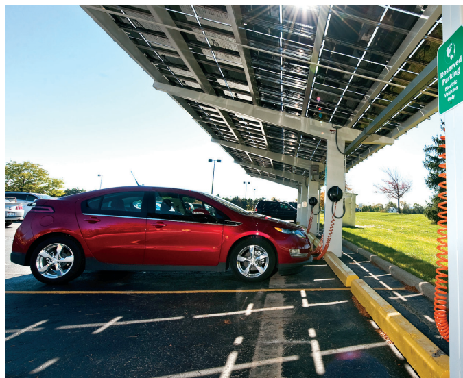
Solar-powered charging stations (such as this one in Detroit, MI) are popping up around the country. Smart charging could enable EVs to draw power from the grid when it is cleanest, and with vehicle-to-grid technology feed surplus clean power back to the grid when electricity demand is higher.
