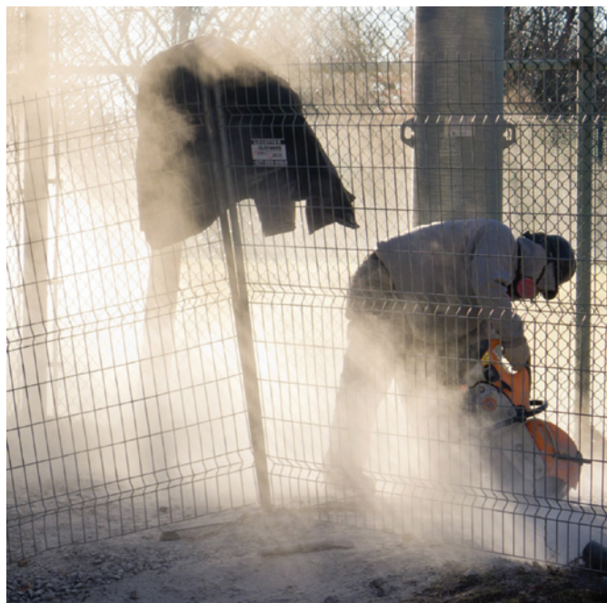
Breathing in the fine dust created when cutting, grinding, drilling, or mining materials containing silica may result in silicosis, making construction workers especially vulnerable to this respiratory disease. In 2013, OSHA proposed new regulations designed to limit workers' exposure, but the ACC has strongly opposed the changes, leaving the proposed rule in legal limbo.
