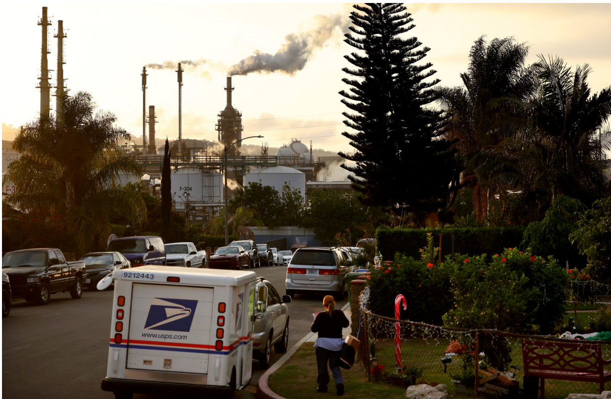
Oil refineries, like this Phillips 66 Los Angeles Refinery in Wilmington, California, expose nearby communities to increased pollution. Closing refineries will alter the future of those communities dramatically. The needs and voices of residents and workers should be central to planning for the transition. Photo: Mario Tama/Getty Images
