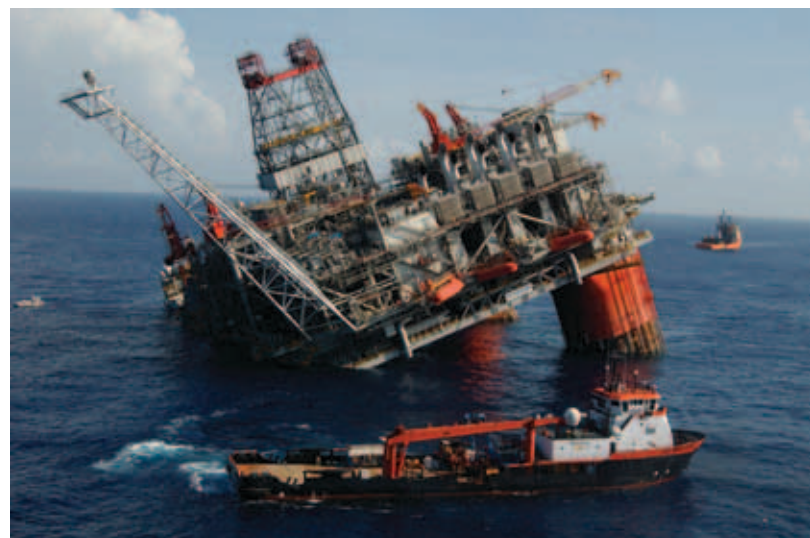
Thunder Horse, an offshore oil platform, damaged in 2005 as a result of Hurricane Dennis. Hurricanes often damage oil and gas infrastructure in the Gulf Coast region, creating gasoline shortages and higher gas prices, particularly in the South.
