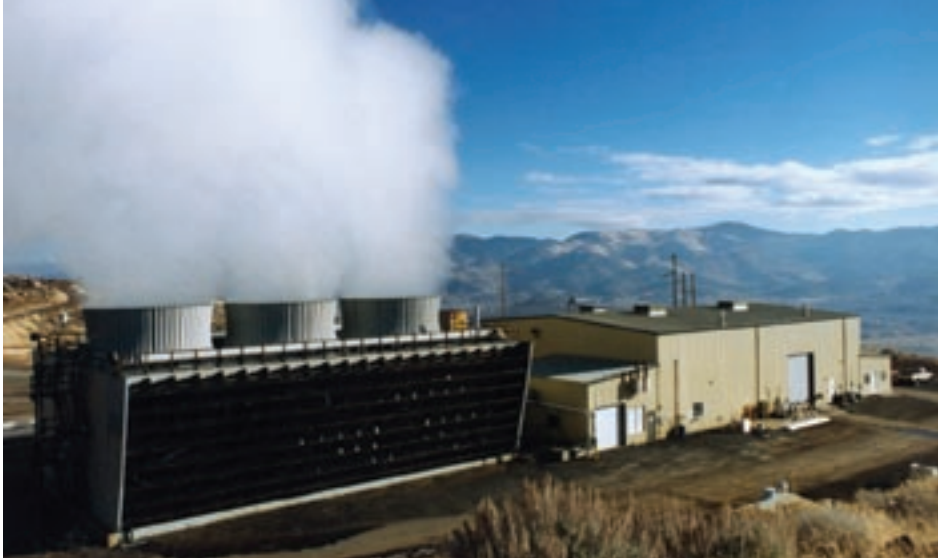
Geothermal power plant. Courtesy of NREL.
