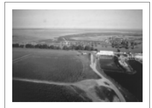
FIGURE 2 Water Control Structure
