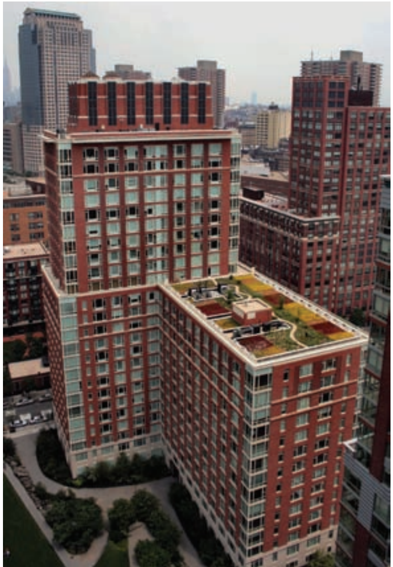
The Solaire apartment building, a 27-story, 293-unit residential tower in Battery Park City, achieved LEED "Gold"-level certification through aggressive goals for reducing energy and water use and peak electricity demand. Completed in 2003, its features include optimal use of daylight, thermal efficiency, high-performance windows, programmable digital thermostats, and Energy Star appliances and lighting fixtures in each unit. Photovoltaic (PV) panels generate 5 percent of the building's peak electricity.
