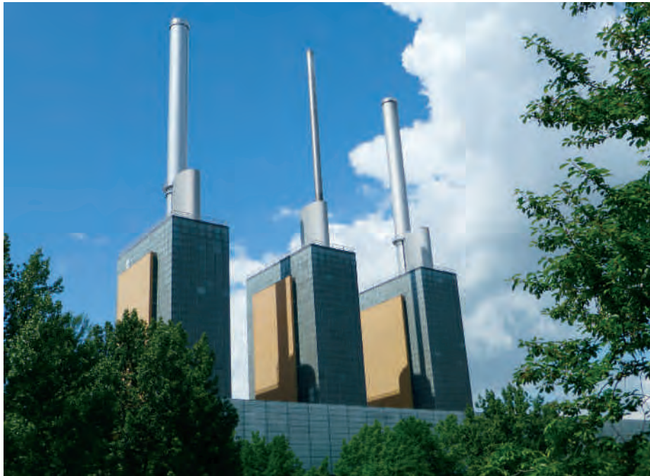
A natural gas combined-heat-and-power plant can provide heating, cooling, and electricity at up to twice the efficiency of the most advanced plant that only generates electricity, while reducing carbon emissions.
