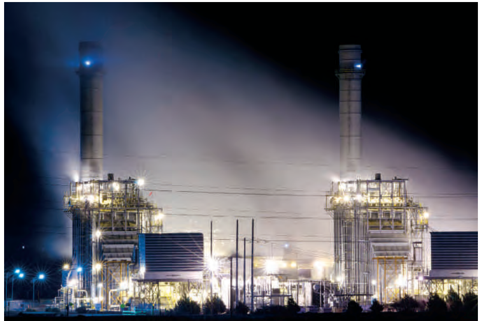
Because of Oregon's strong renewable energy policies and its abundant wind resources, this natural gas combined-cycle plant in Hermiston now operates as a balancing plant to complement the area's recent growth in wind power.
