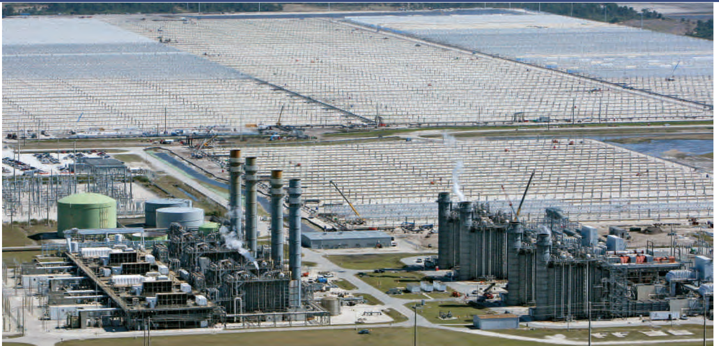
Florida's overreliance on natural gas—for more than two-thirds of its electricity generation in 2012—makes its economy vulnerable to price spikes. The use of solar energy at the Martin Integrated Solar Combined Cycle plant located in Indiantown, Florida (which combines concentrating solar power with natural gas power generation), will help reduce this vulnerability, but the Sunshine State is still far behind the rest of the country in investing in renewables and energy efficiency (Cleetus et al. 2012).
