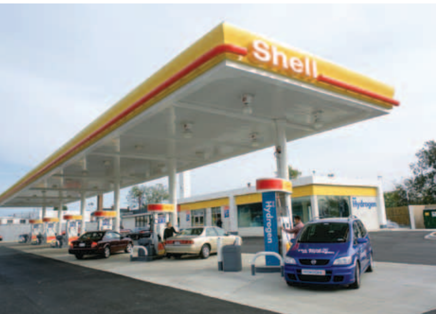
Shell Hydrogen and General Motors teamed up to build the first combined hydrogen and gasoline fueling station in North America, located in Washington, DC.
