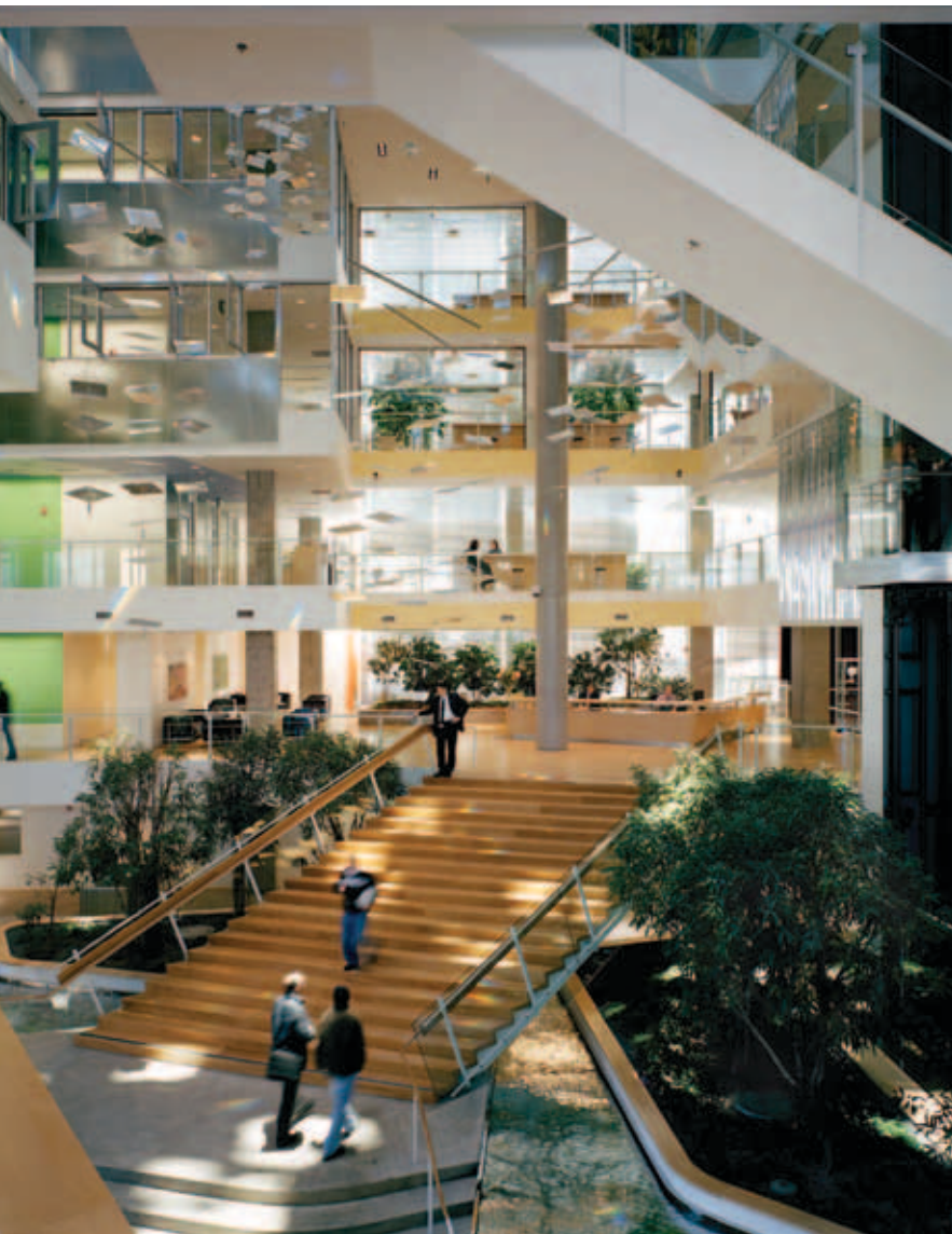
By incorporating efficient design features and building materials, the LEED Platinum-certified Genzyme Center in Cambridge, MA, reduces its energy costs by more than 40 percent compared with a comparable building. Heat-retaining concrete slab construction moderates the interior temperature, while a double-paned glass curtain wall maximizes insulation and allows most employees to work in naturally lit space. Genzyme benefits from reduced energy costs while employees enjoy the improved quality of their work environment.
