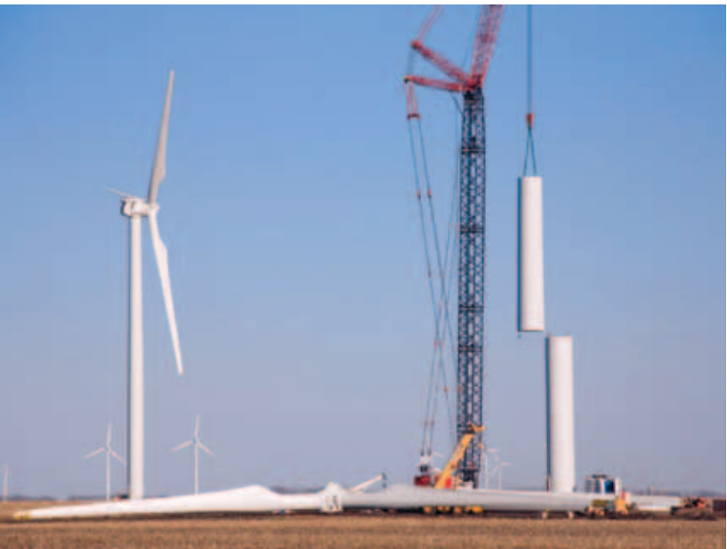
Climate 2030 Blueprint policies will benefit the U.S. economy by spurring investments in clean energy technologies and saving consumers and businesses money—in every region of the country.
