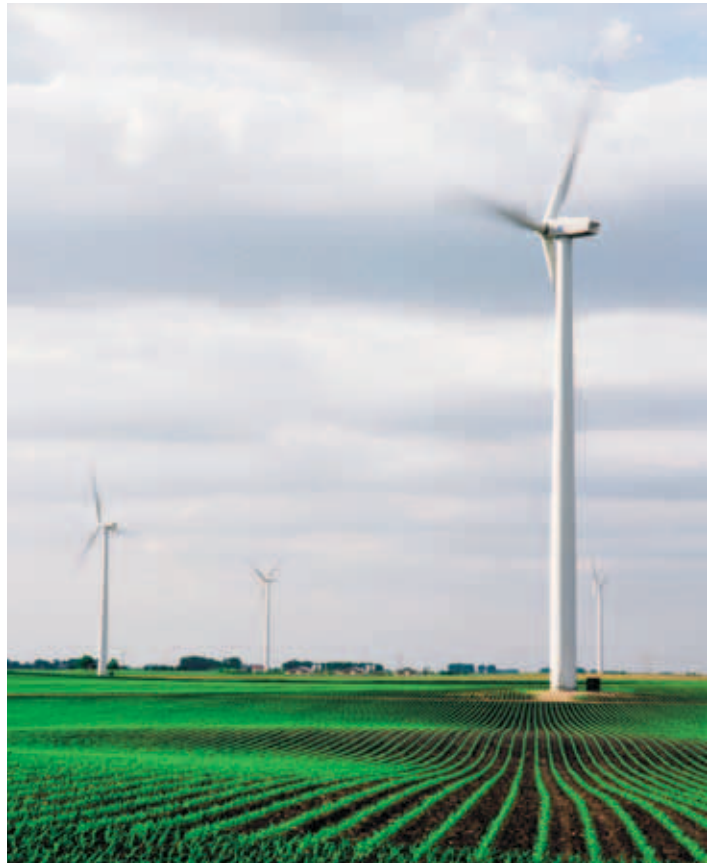
Wind power can provide an important economic boost to farmers. Large wind turbines typically use less than half an acre of land, including access roads, so farmers can continue to plant crops and graze livestock right up to the base of the turbines (as shown on this Trimont, MN, farm).
