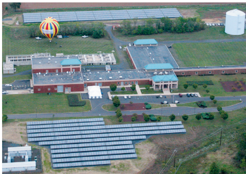
© NJ Board of Public Utilities
