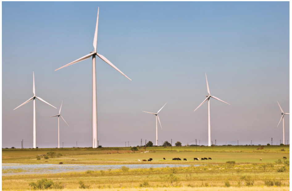
These wind turbines, on a West Texas farm near McAdoo, are part of the tremendous effort to develop the state's vast wind resource. As of the end of 2012, more than 12,000 MW of wind capacity had been installed in Texas, making it the leader in wind development in the United States.
