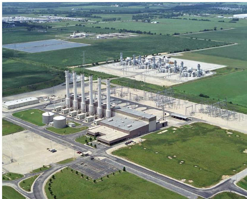
Reducing energy demand can avoid the use of expensive "peaking" plants (like the Woodsdale natural gas plant in Butler, OH, above).
