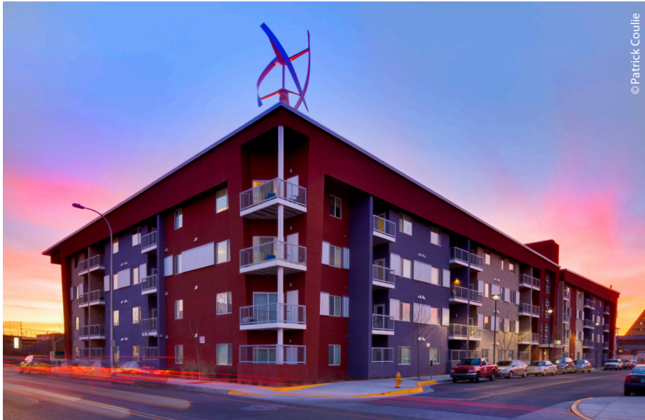
The Silver Gardens Apartments in Albuquerque, NM, which provide homes for residents with a mix of incomes in a transit-accessible location, include energy-saving design features that make the apartments 40 percent more efficient than conventionally built counterparts.
